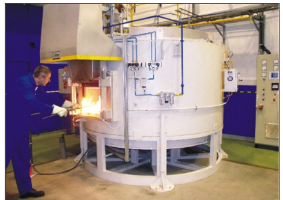
Furnaces with manual loading system
