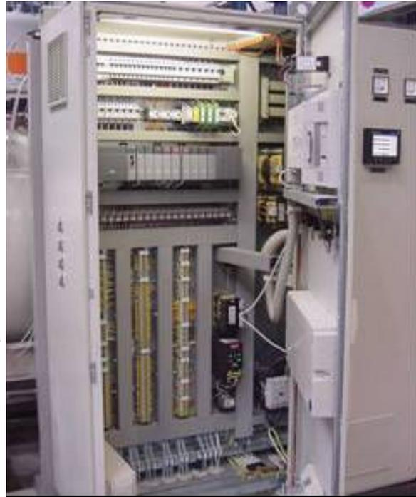
The furnace operating sequence is written in a form of a program in the Central Processing Unit (CPU) of the controller and is stored in the non-volatile memory.
